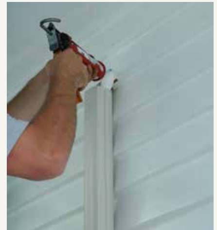
b. Applying sealant around pipework.
