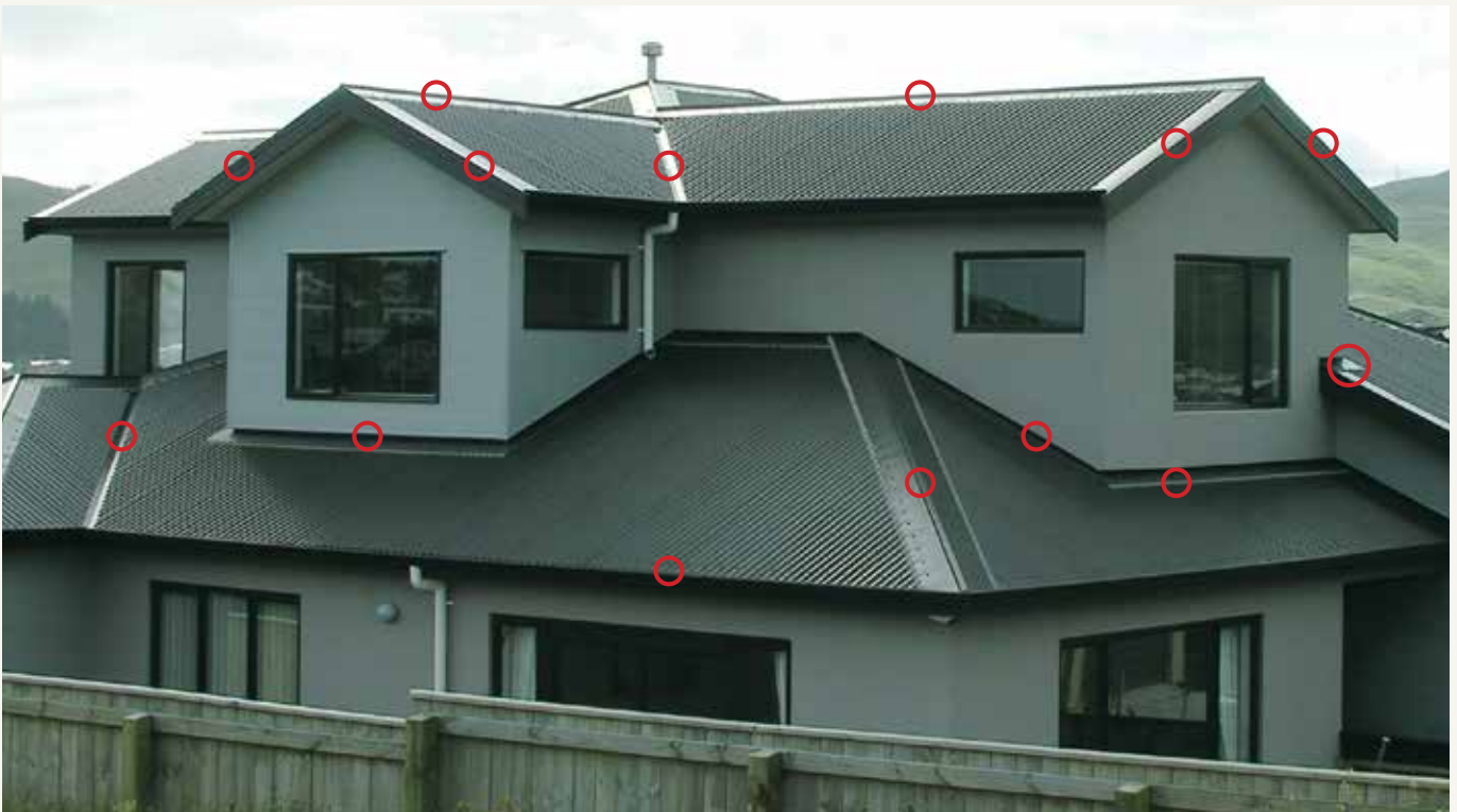
Junctions where flashings are required.
