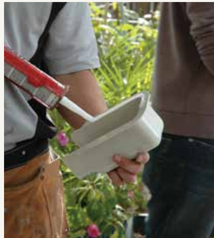
c. Applying sealant to cover.
