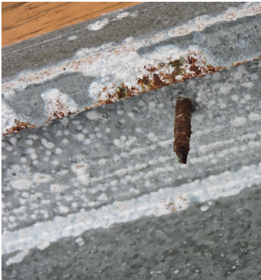
Figure 3: A closer view of the rust on the hold-down screws in the galvanised purlin in Figure 2.
