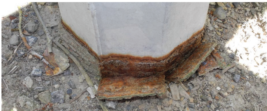
Figure 1: Ring bark corrosion on 18-year-old lighting pole. This has lost up to 40% of its original thickness.
