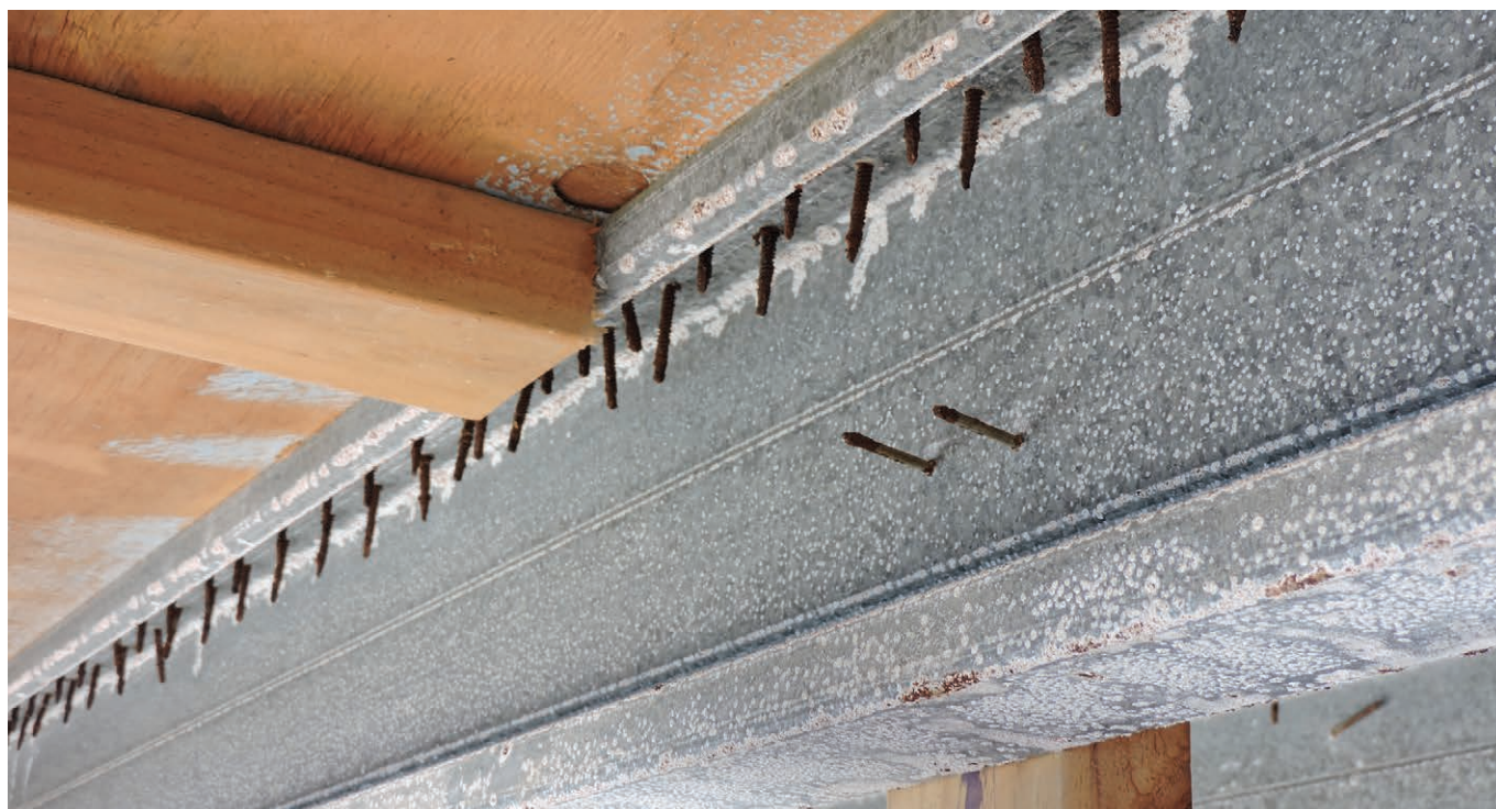
Figure 2: Roof cavity in 1990s house. Inline galvanised purlins with a heavy build-up of white and red rust indicating depletion of the original corrosion protection.
