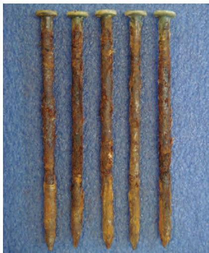
Figure 4: Galvanized steel nails embedded into H4 ACQ treated timbers exposed at Judgeford for 3 years. The condition of the zinc coatings on the head and the body were significantly different.
