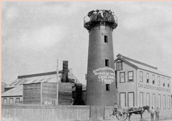
East Cape Lighthouse (1900) made in cast iron by the Thames Iron Works. (Source: Cyclopaedia of NZ Vol. 2, Auckland 1902.)
