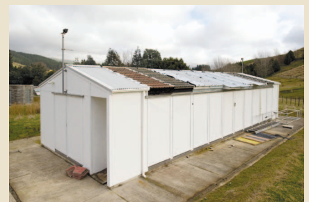
Figure 1: BRANZ multi-roof test building.
