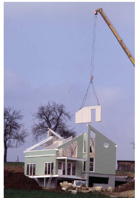
A fully closed wall element is positioned by crane. (Source: Baufritz.)
