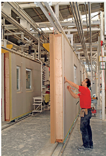
Operator finishes a fully closed timber-framed wall panel. (Source: Weberhaus.)
