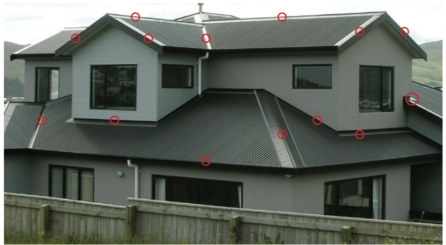
Junctions where flashings are required.
