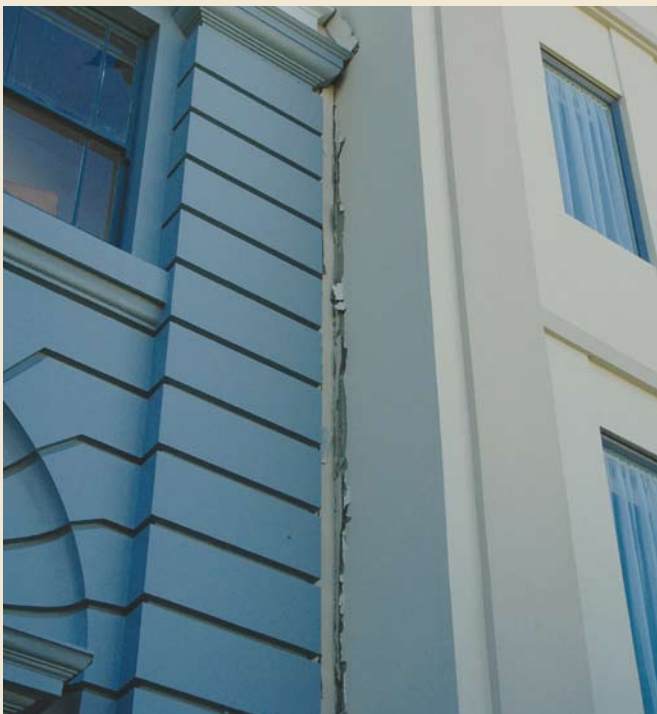
Damage in Gisborne from pounding of adjacent buildings.
