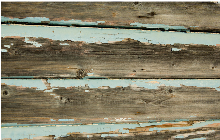
Where the paint is in poor condition, it may be best to strip it back to bare timber and repaint.
