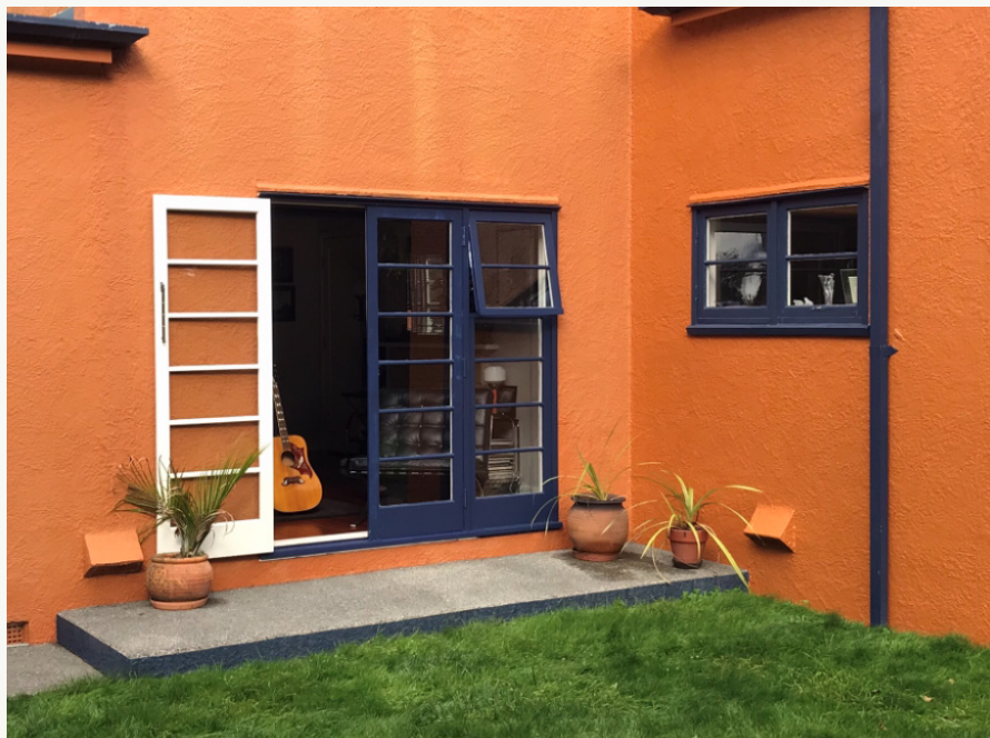
A period-style timber doorset replaced an original window, transforming the liveability of this period home.
