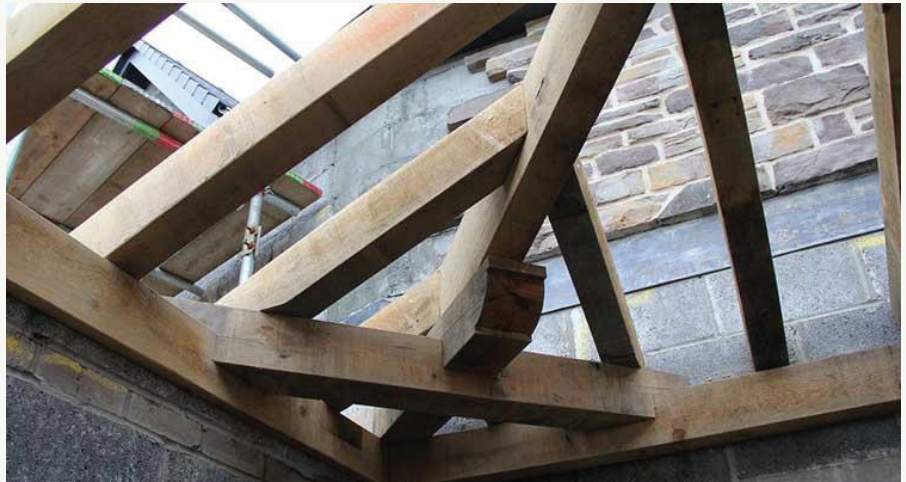
Figure 1 Traditional dragon tie arrangement in heavy roof construction.
