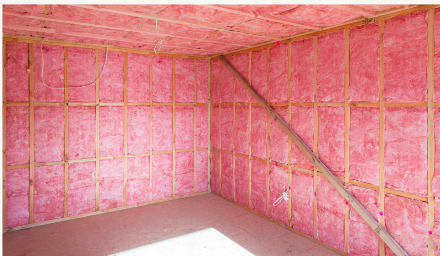
Higher R-value insulation combined with reducing excess framing is a cost-effective way of improving the performance of the thermal envelope.
