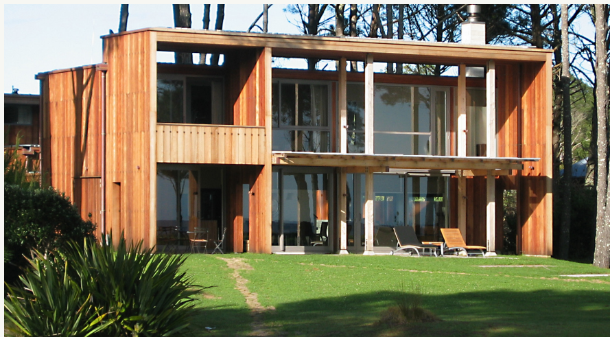
Consideration should be given to extent and orientation of glazing, as well as shading to ensure homes don't overheat during warm months.
