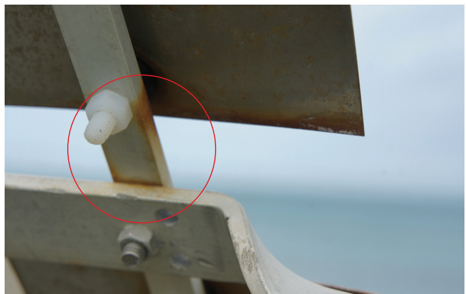
Figure 3. Stains on aluminium due to water run-off from a corroding stainless steel (grade 304) surface in a severe marine environment.
