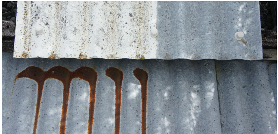
Figure 1: Water run-off from a prepainted steel surface can damage galvanized steel installed underneath.
