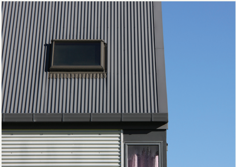
Long-run metal roofing.
