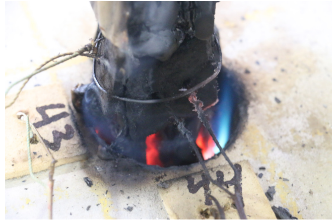
Figure 2: A failed cable penetration in the timber infill floor test – no firestopping had been applied to this penetration.
