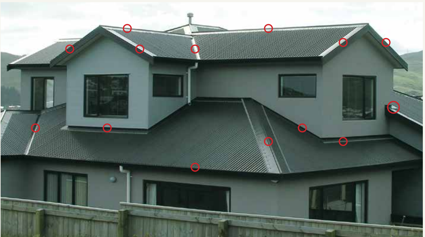
Junctions where flashings are required.
