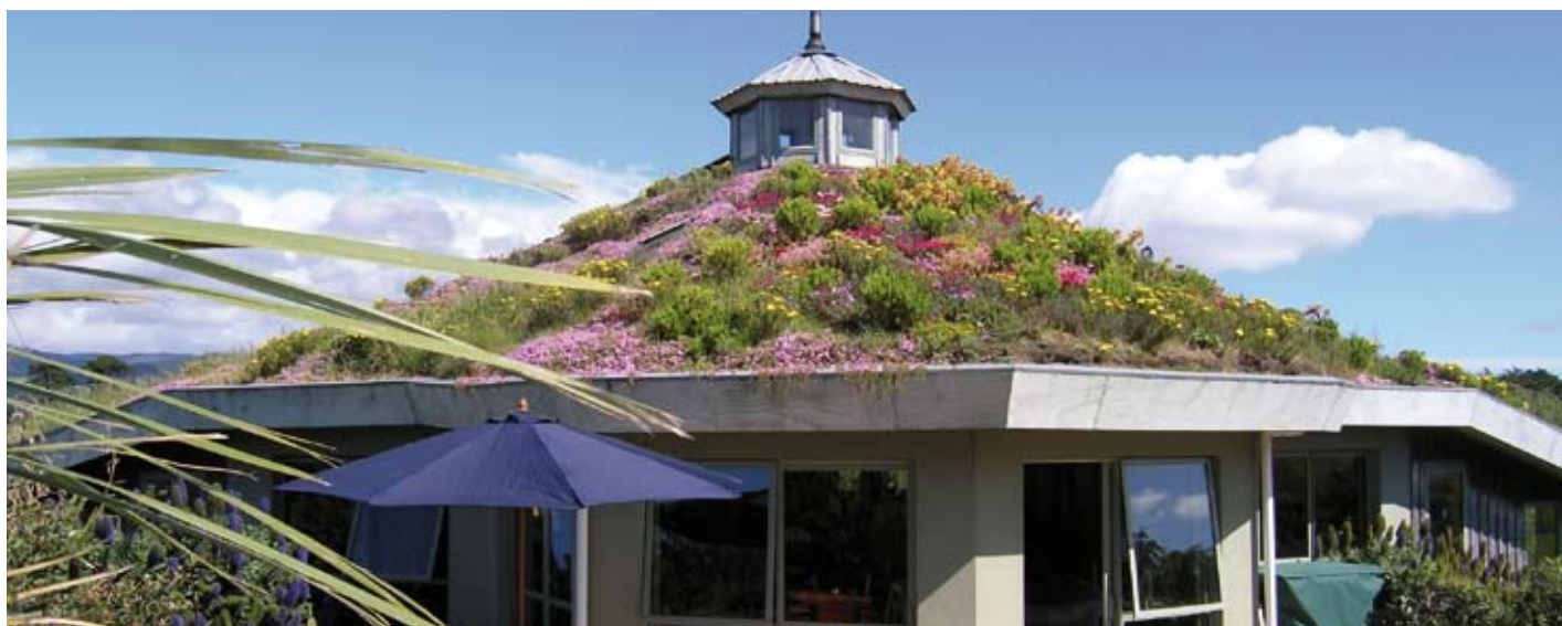
Established green roof on a house in Kapiti during summer. The plants are mostly New Zealand iceplant. (Photo by John Le Harivel, Architect.)
