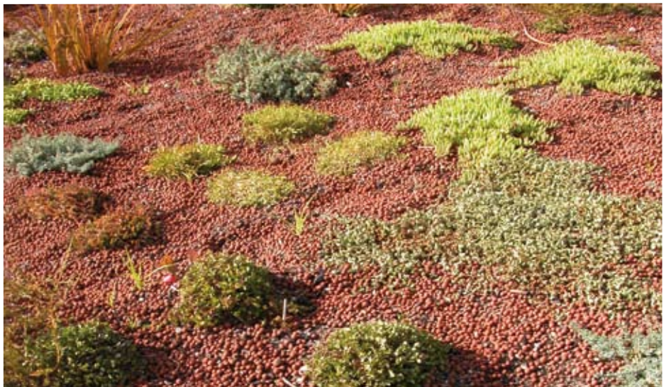
3. The completed roof with native plants in expanded clay planting medium. (Photos from Waitakere City Council.)
