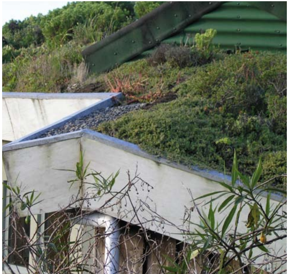
Detail of the gravel gutter which has a perforated land drain laid to fall to outlets. (Photo by John Le Harivel, Architect.)
