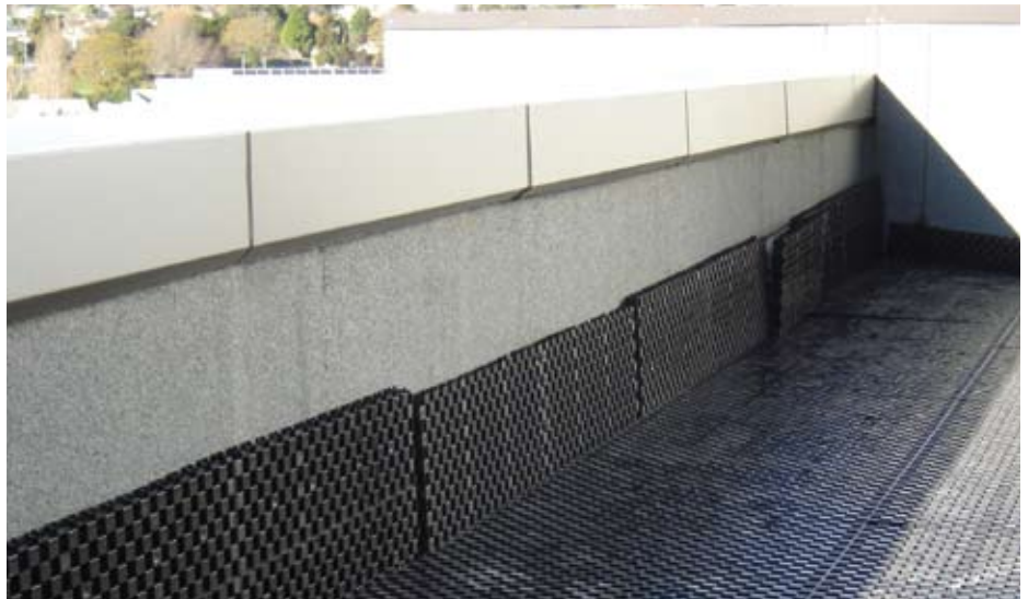
Construction of the green roof at the Waitakere City Council Civic Centre. 1. The drainage cell layer is placed on the roof area.
