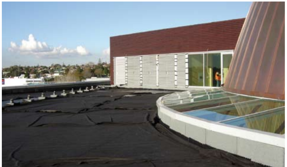
2. The geotextile fabric is ready for the growing medium.
