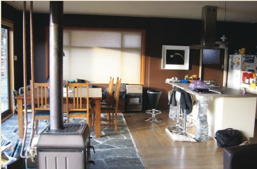
The living room, showing alterations such as the stone floor, north facing window and thermal blinds.
