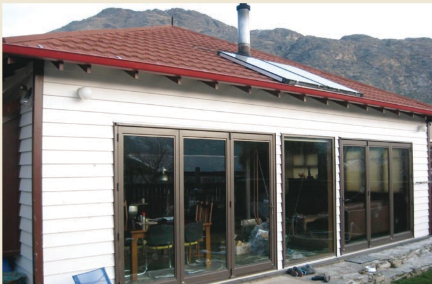
The living room, showing alterations such as the stone floor, north facing window and thermal blinds.
