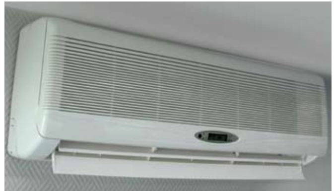
Most heat pumps in New Zealand are air source heat pumps like this one.
