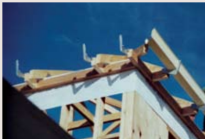
Stages in the installation of a concealed guttering system.
