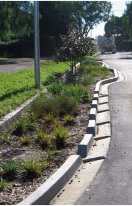
Rain gardens within the new public road.
