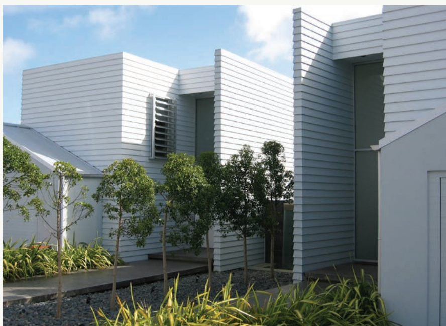
Modern interpretation of timber weatherboards.
