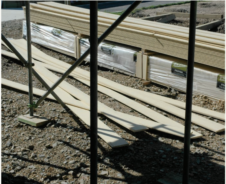
Poor storage and handling is commonly observed on site.
