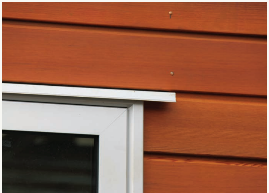
Windows aligned with the board set-out.
