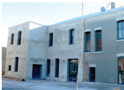
Figure 10: Retrofit with shotcrete on the rear of a building.
