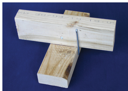
Figure 1: Type E fixing used in NZS 3604:2011 is always 2 skew nails plus 2 wire dogs in this configuration.
