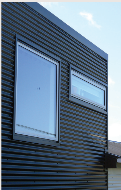
Figure 1: The lack of eaves means that the wall will be rain-washed but the weathertightness risk that has to be designed for is higher.
