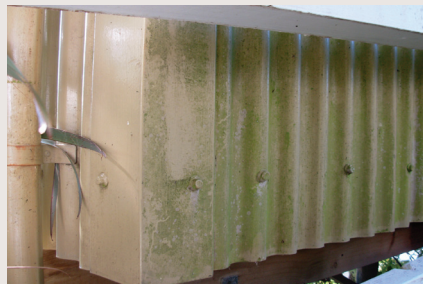
Figure 3: Moss growth on painted profiled metal cladding due to lack of cleaning.
