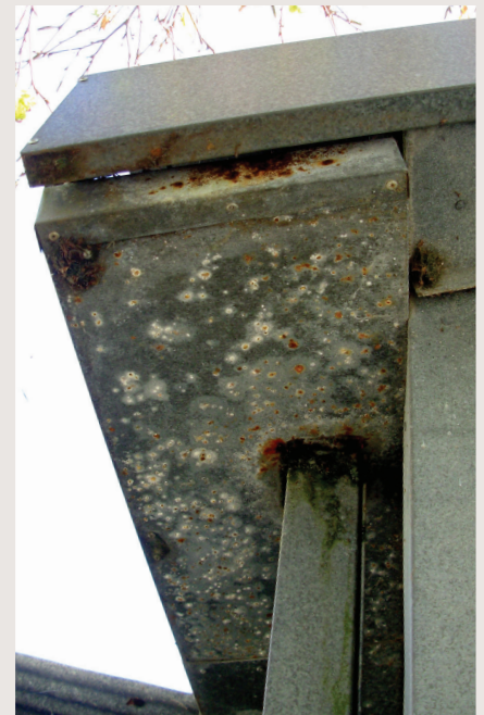
Figure 4: More severe red and white rust corrosion on the underside of a metal gutter where it has not been rain washed or cleaned.
