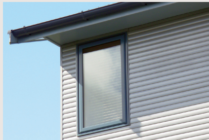
Figure 2: Aluminium weatherboard wall cladding. The top of the wall will not be rain washed and will require cleaning.
