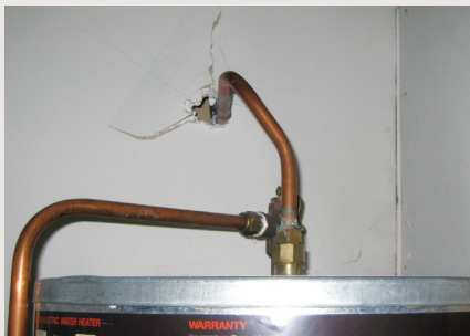
Figure 1: Damage to wall linings from unrestrained hot water cylinder.
