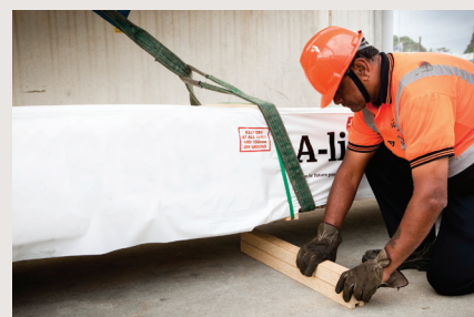
Unload boards by hand if there is no mechanical equipment available. (All photos courtesy of Jenkin Timber Limited.)
