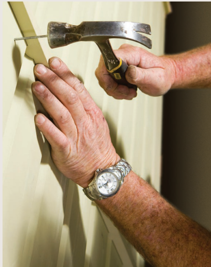
Hand nailing is recommended with only one nail per board at each stud spacing.
