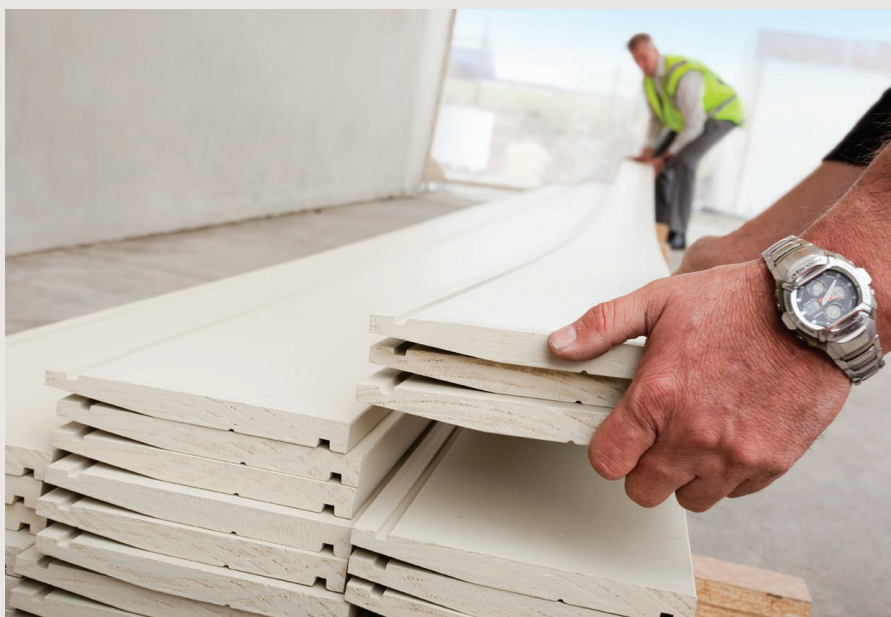
Unload boards by hand if there is no mechanical equipment available. (All photos courtesy of Jenkin Timber Limited.)
