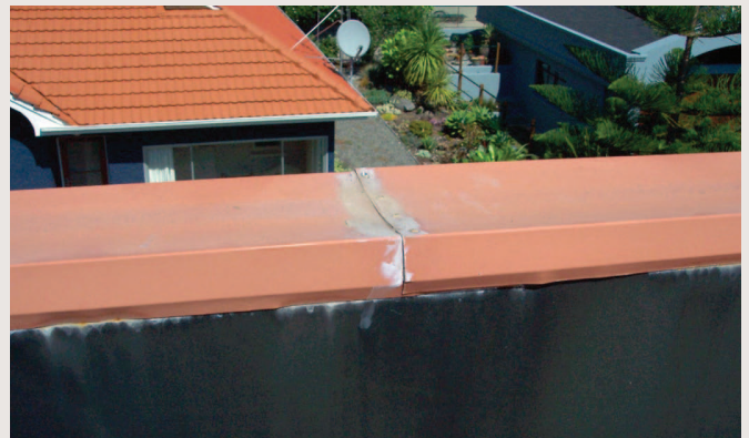
Figure 6: Incorrectly sealed and lapped cap flashing joint. Water has entered through the sealant lap and riveted fixings. The flashing overlap is too small and is dished from lack of support.
