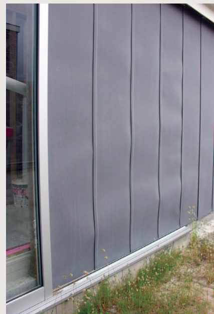
Figure 1: Material that has its movement restricted and can not expand or swell freely will buckle or split, like this zinc panelling.
