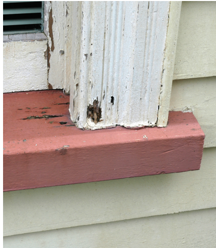
Figure 2: Rot in the sill and facing resulting from water being trapped in the joints and being absorbed into the timber.
