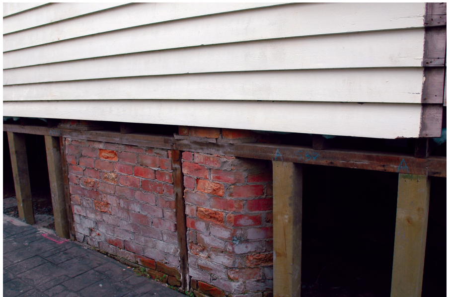
Figure 1: Moisture can be seen rising up through the base of this chimney brickwork. The height of the brickwork minimises the risk of moisture damage to framing.
