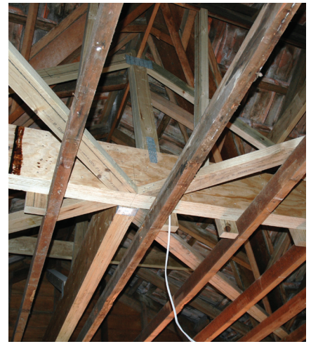
Figure 5: Trussed strongback supporting ceiling joists.
