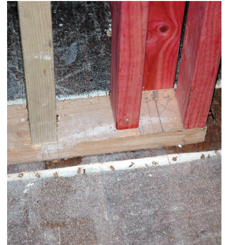
Figure 3: Staggering the new internal wall framing at an external wall corner to accommodate the smaller new framing and allow for the fixing of new linings.
