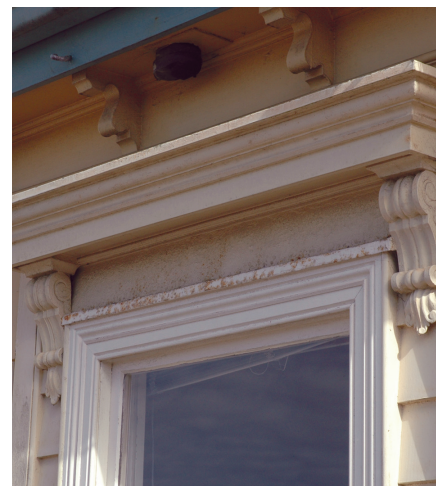
Figure 7: Corrosion of head flashing.
