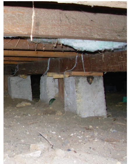
Figure 6: Replacement precast concrete piles with wire ties to the bearers. Original timber piles are also visible.
