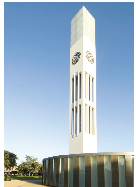
Hopwood clock tower before refurbishment (top) and afterwards (bottom).
