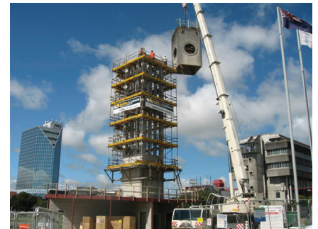
Replacing the renovated lantern section.
