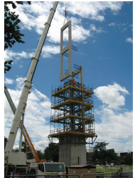
Precast sections being put in place.
