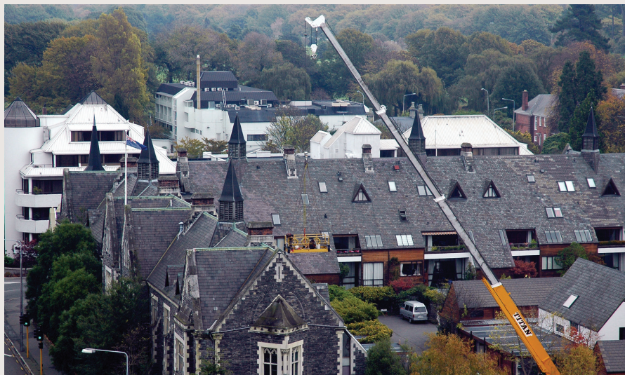
Not all roofs were designed with maintenance in mind.
