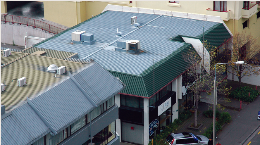
Recoating was only carried out on those parts of the roof visible from the street.
