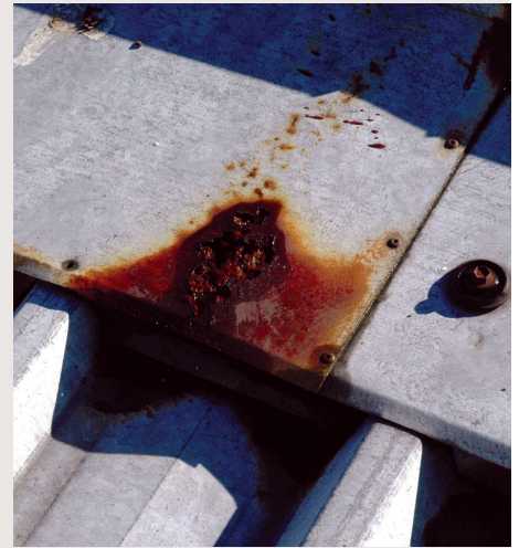
Corrosion is an ongoing risk with an unpainted galvanised steel roof cladding in an industrial environment.
