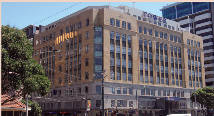
Tower Insurance building, Wellington (previously known as Government Life), built in 1931.
