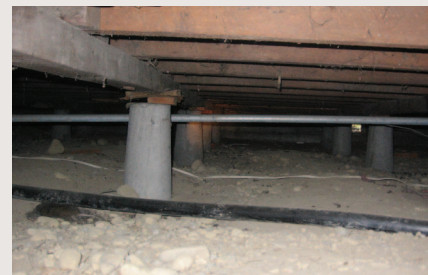
Figure 2: Many piles are not connected to the floor framing.
