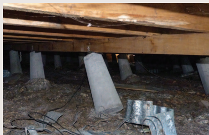
Figure 1: Piled foundations that moved during the Darfield earthquake.
