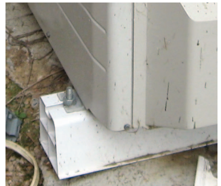
Figure 2: Unit not fixed to the ground.
