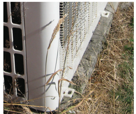
Figure 3: No clearance under the unit.
