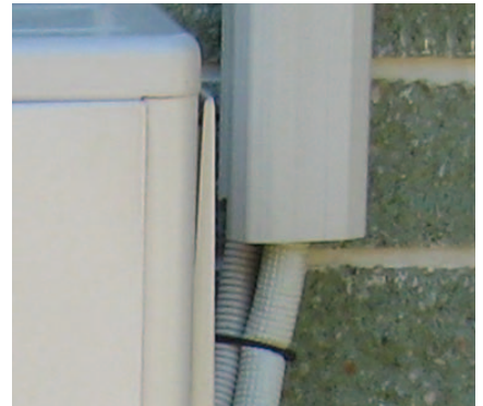
Figure 1: No sealant in the gap at the end of the ducting.
