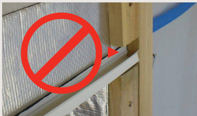
Figure 3: How not to install a Wanz-WIS cavity drain over a window.
