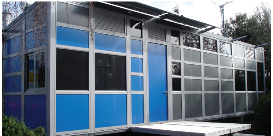
The HABODE prefabricated design includes sustainable features such as double glazing and thermal insulation. (Photo: Pamela Bell.)
