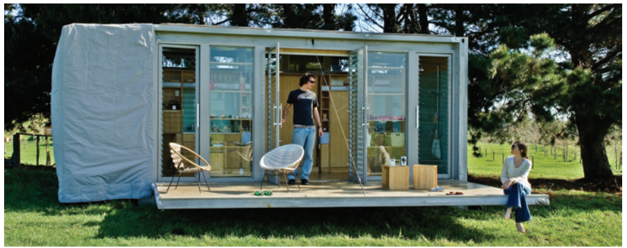
Atelier Workshop's port-a-bach design features a fold-down deck that refolds to create a secure unit for insitu storage or relocation. (Photo: Paul McCredie.)
