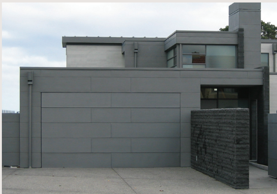
Large metal garage doors can be a significant source of heat loss and air leakage when the garage is included within the thermal envelope of the building.
