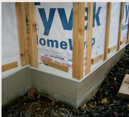
Figure 1: The horizontal timber correctly has gaps and is sloped to allow water through but there should be a gap between corner battens (see Figure 2).
