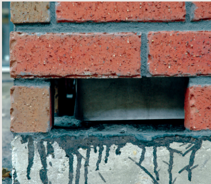
View through a clean-out opening showing a typical masonry veneer rebate, that accommodates a 70 mm wide brick and a 50 mm wide cavity between the foundation edge and the step at the base of the structural frame. Note the wall underlay is too close to the rebate.
