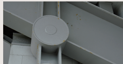
Access is readily available to recoat the face of the steel shown, but what about the coating durability on the rear face, which appears relatively inaccessible?
