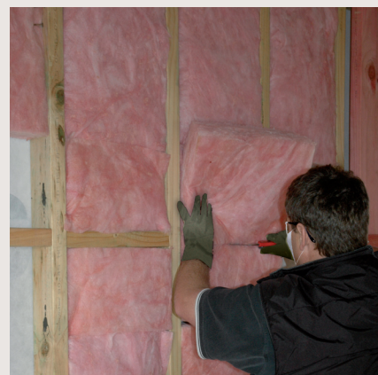
Press the material into place without creasing, folding or compressing it.
