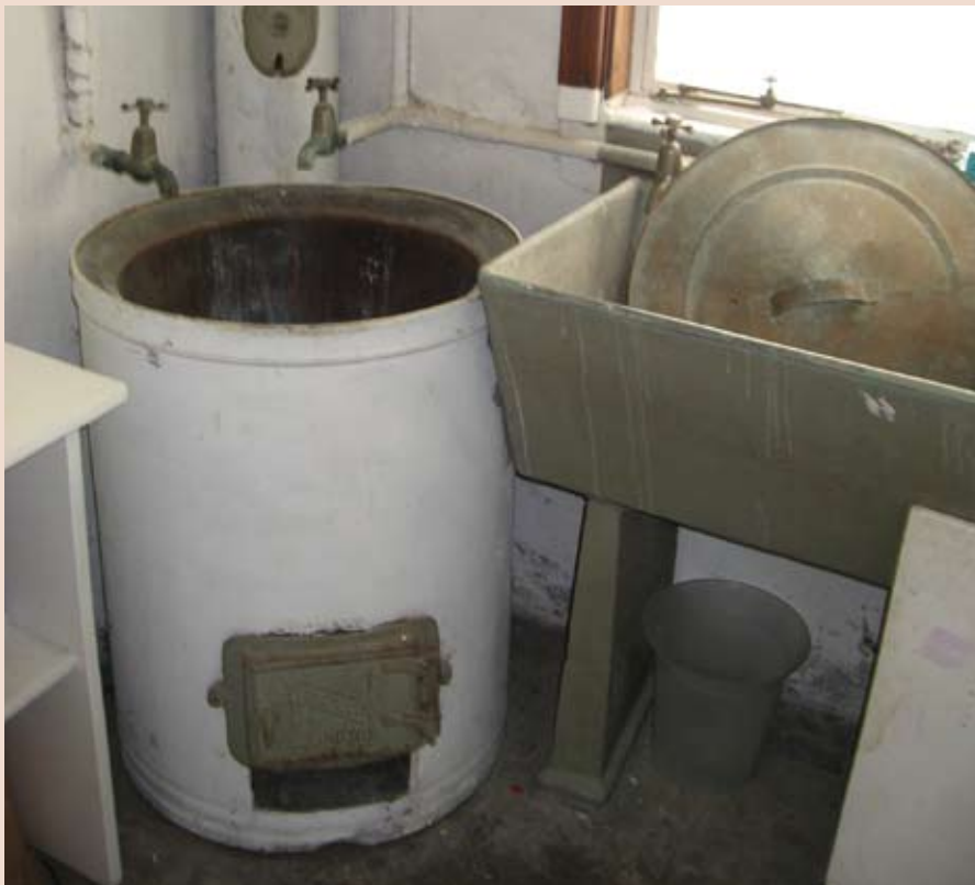
A 1930s laundry copper with piped hot water. Note the firebox cover below and the flue cleaning slot.
