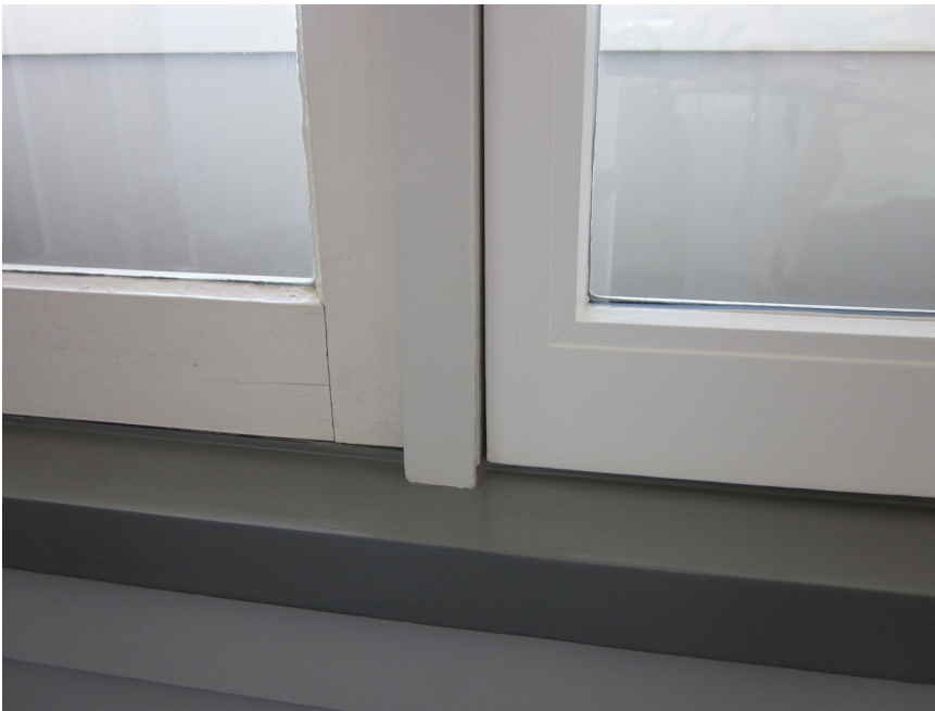
Figure 2: Comparison of casement windows with single glazing (left) and retrofitted IGU (right).
