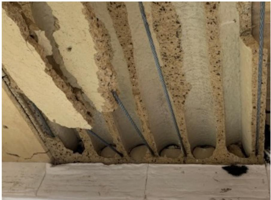
Figure 2: Damage to the underside of the floor after the fire experiment. Close-up in the bottom photo.
