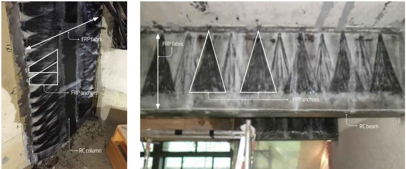
Figure 1: Examples of the use of fibre-reinforced polymer (FRP) anchors.
