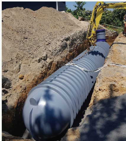
Underground retention and detention system. Photo courtesy of Hynds.
