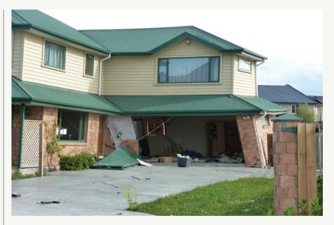
Extensive damage to a light timber-framed house following the Canterbury earthquakes.
