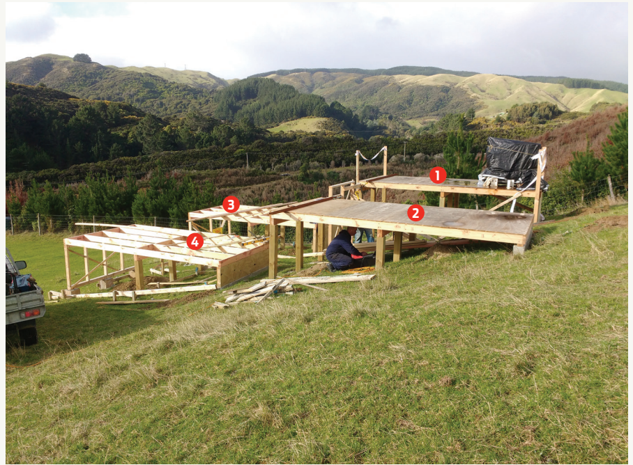
Figure 2 Test foundations being built – NZS 3604:2011 floors 1 and 2 on the right and pre-1960 floors 3 and 4 on left.
