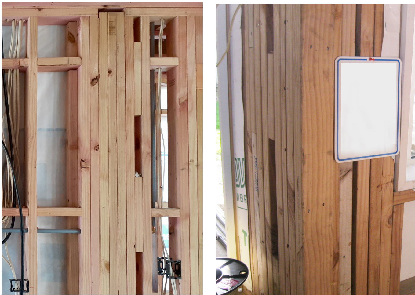
Figure 1: Case study houses with a very high percentages of wall framing (left) and corner framing (right). These areas of walls will be almost completely uninsulated.
