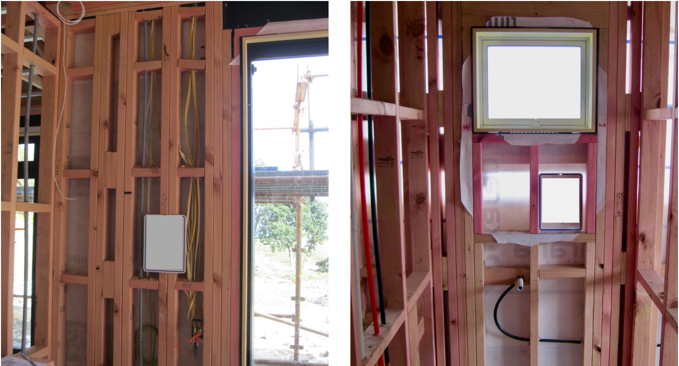
Figure 2: Although built to the Building Code, the high percentage of wall framing from close nogging, blocking and multiple studs next to a large window (left) leaves little space for insulation. The small toilet wall (right) is an area prone to condensation, but insulation will only be able to fit in a small percentage of this wall.
