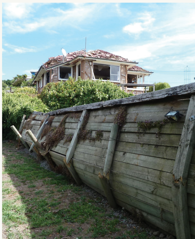
Failed timber retaining wall following earthquakes.
