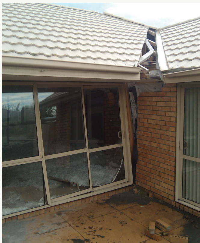
Damage from liquefaction following the Canterbury earthquakes.
