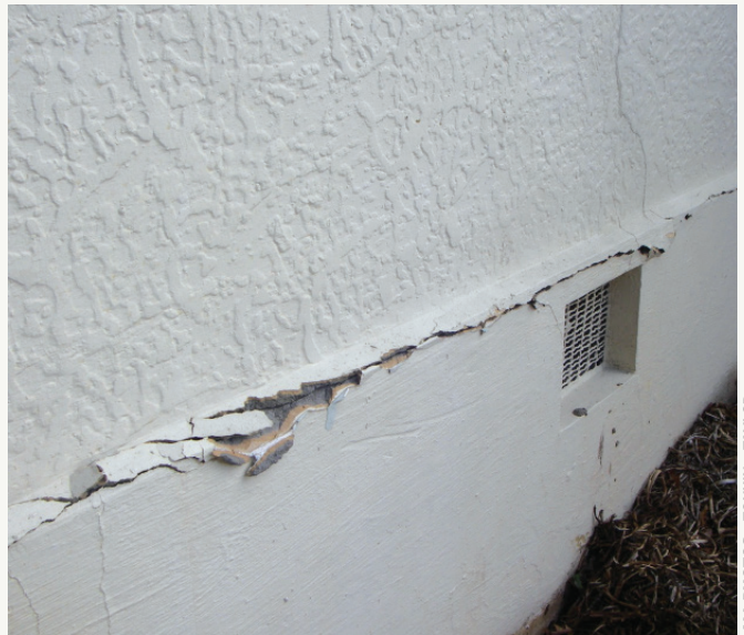
Damage from ground shrinkage and settlement following a drought.
