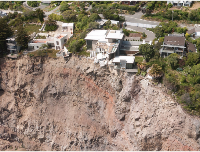
Earthquake shaking displacing cliffs and severely damaged buildings.
