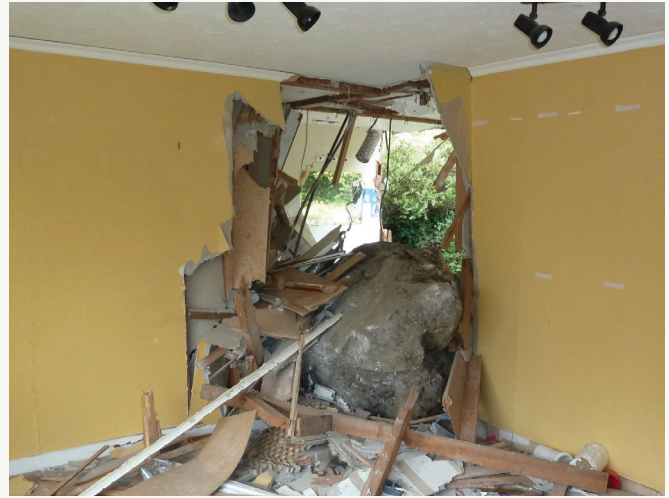
Damage from a boulder dislodged during an earthquake.
